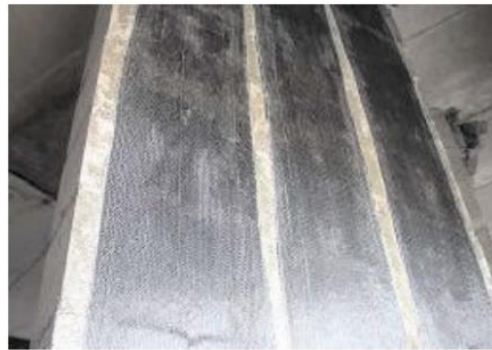
Figure 2-16. Retrofit setup (Urgessa and Maji, 2010)
