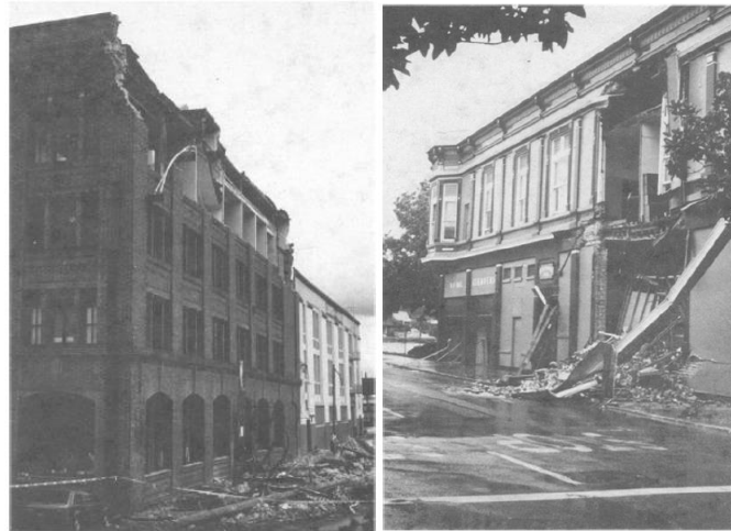
Figure 2-4. Examples of Out-of-plane failure of URM walls caused by earthquakes (Bruneau, 1994)
