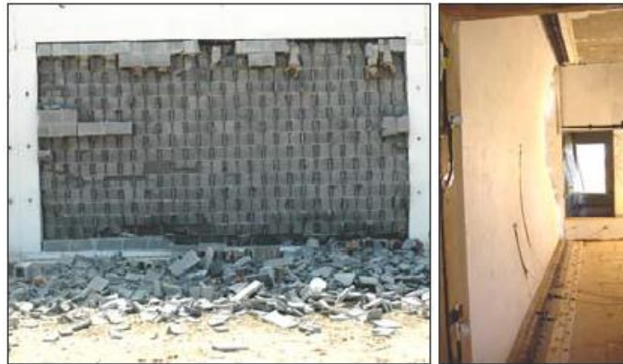
Figure 2-27. Results of wall retrofit with spray on polyurea. (Johnson et al., 2004)
