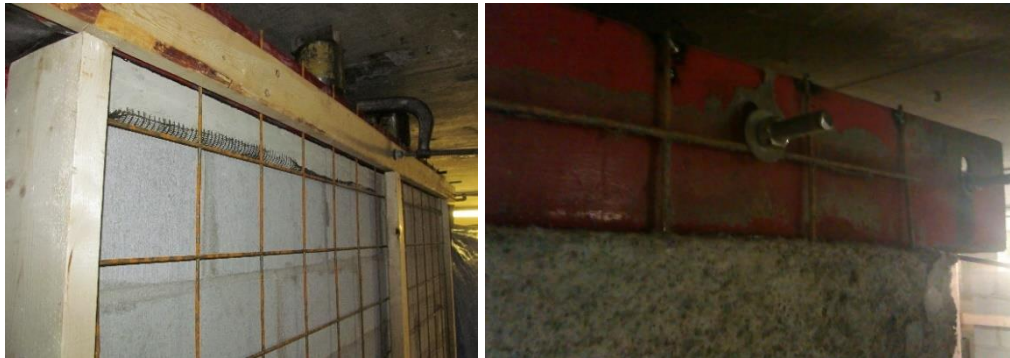
Figure 3-10. Before and After shotcrete was applied.
