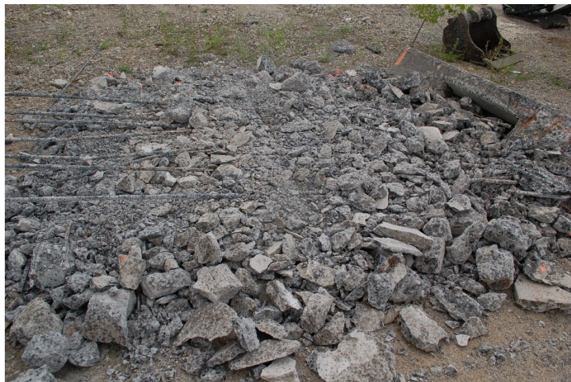
Figure B.0.7: Slab 14 After Rebar Removed
