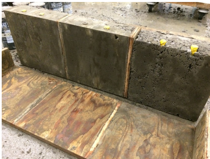
Figure A.0.3: Formwork Removal
