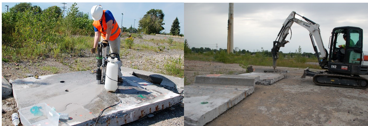
Figure 3.24: Field Study – Cornwall Destructive Testing
