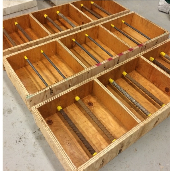
Figure 3.9: Completed formwork ready for concrete pouring
