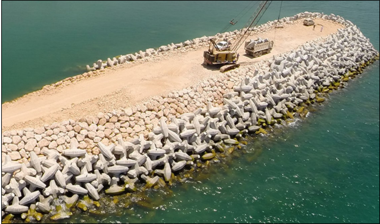
Figure 2-7: Core-loc breakwater under construction (CLI, 2012)
