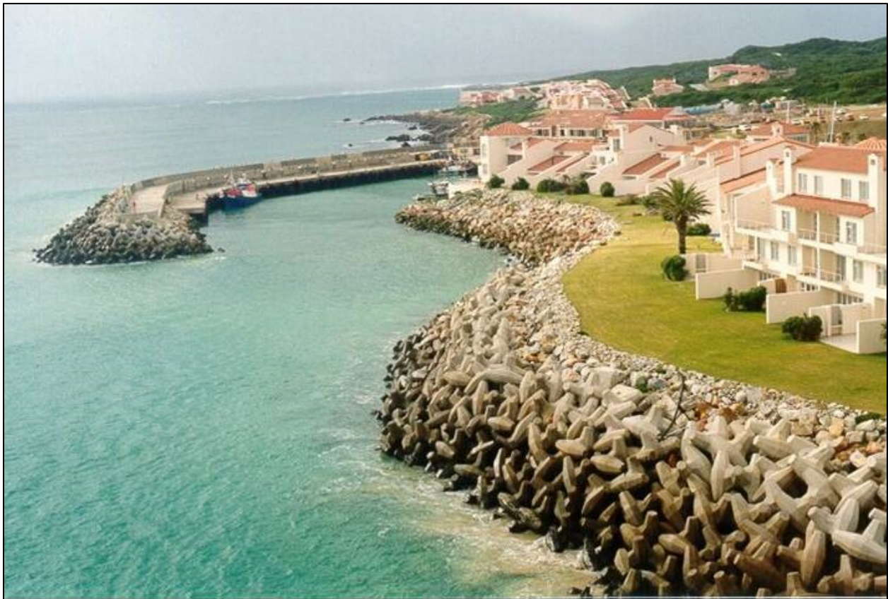
Figure 1-1: Shore connected breakwater and rubble-mound revetment, Port St. Francis, South Africa 1
