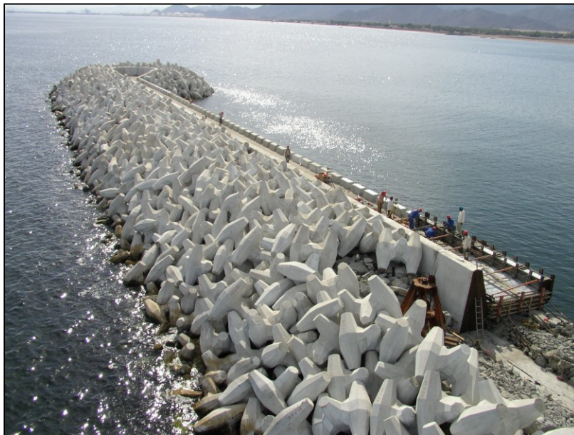
Figure 2-1. Breakwater under construction using Core-loc single layer system 2
