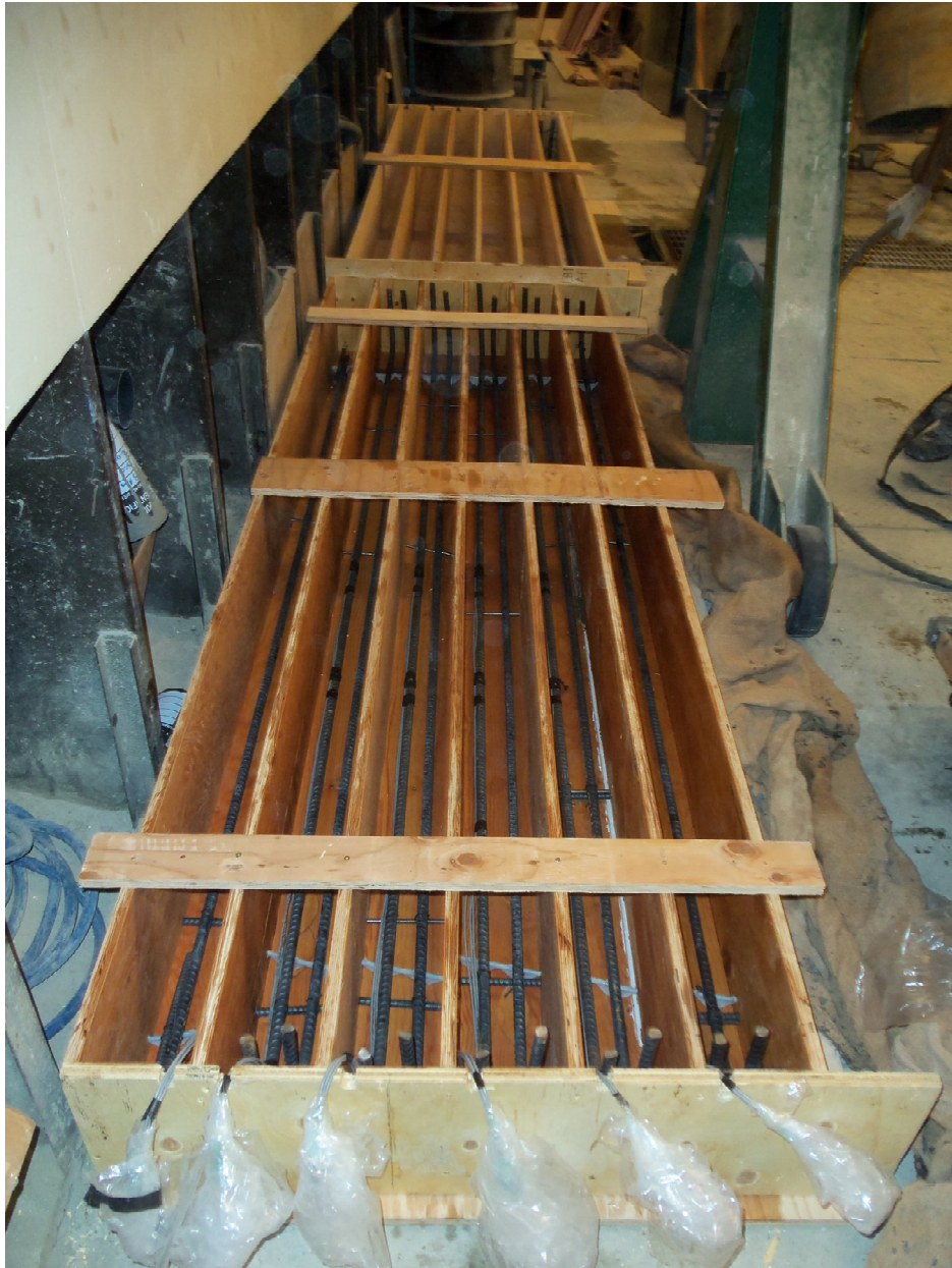
Figure 3.6: The form work used to cast all the beam specimens
