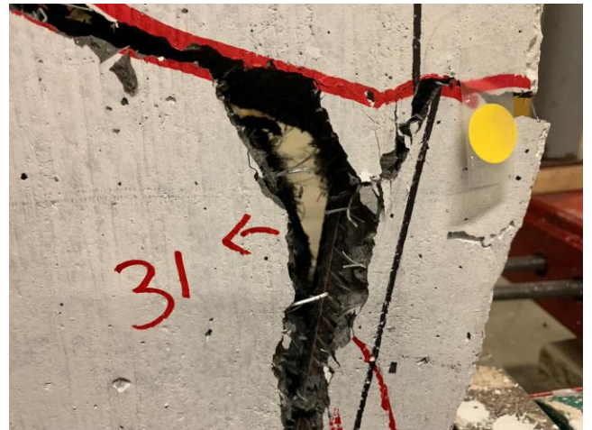
e) Principal shear crack (Blast 2a)
