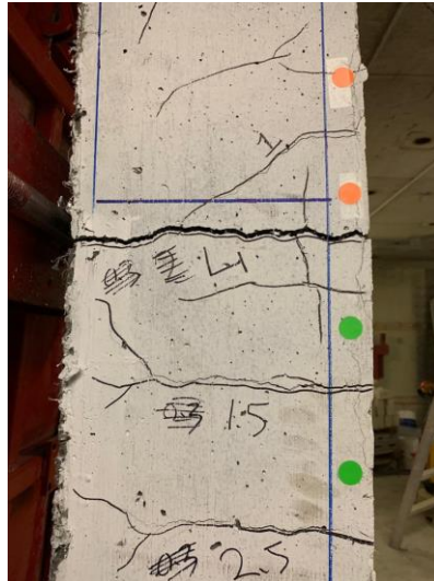
f) Crack propagation (Blast 2c)
