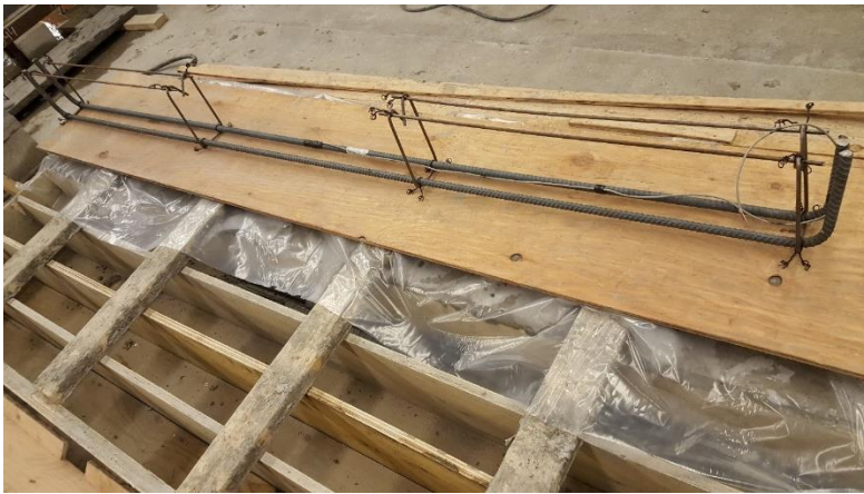
Figure 3-12 15M rebar without stirrups
