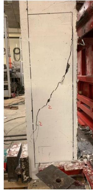
b) Close-up of shear failure (Blast 1)
