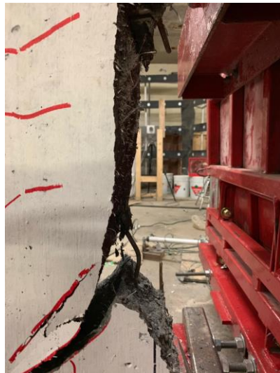
d) Failure close-up (Blast 2a)
