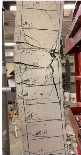
e) Concrete crushing (Blast 3b)
