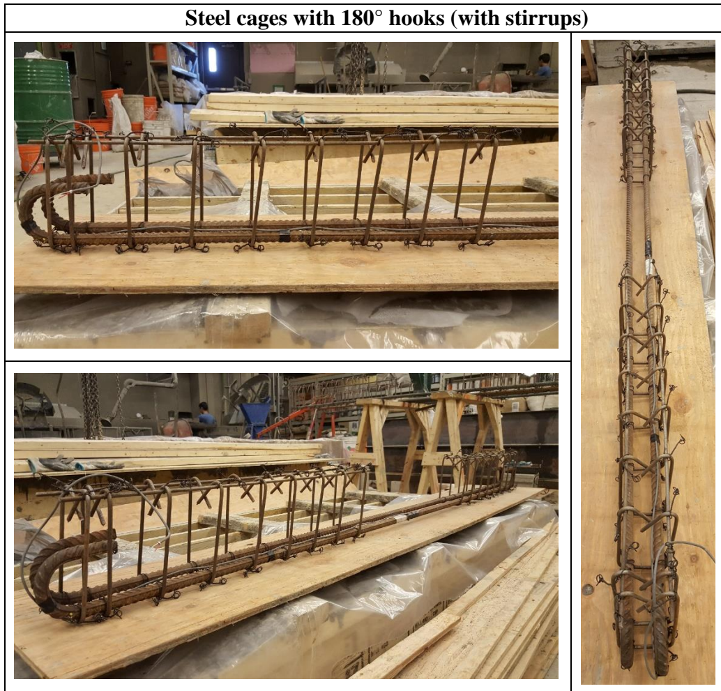
Figure 3-15 20M rebar with stirrups
