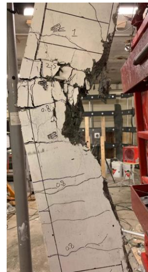
g) Concrete crushing & fiber pullout (Blast 3a)
