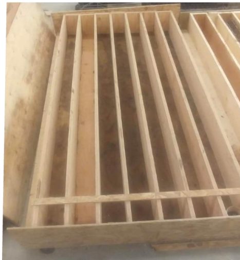
Figure 3-10 Beam wood formwork
