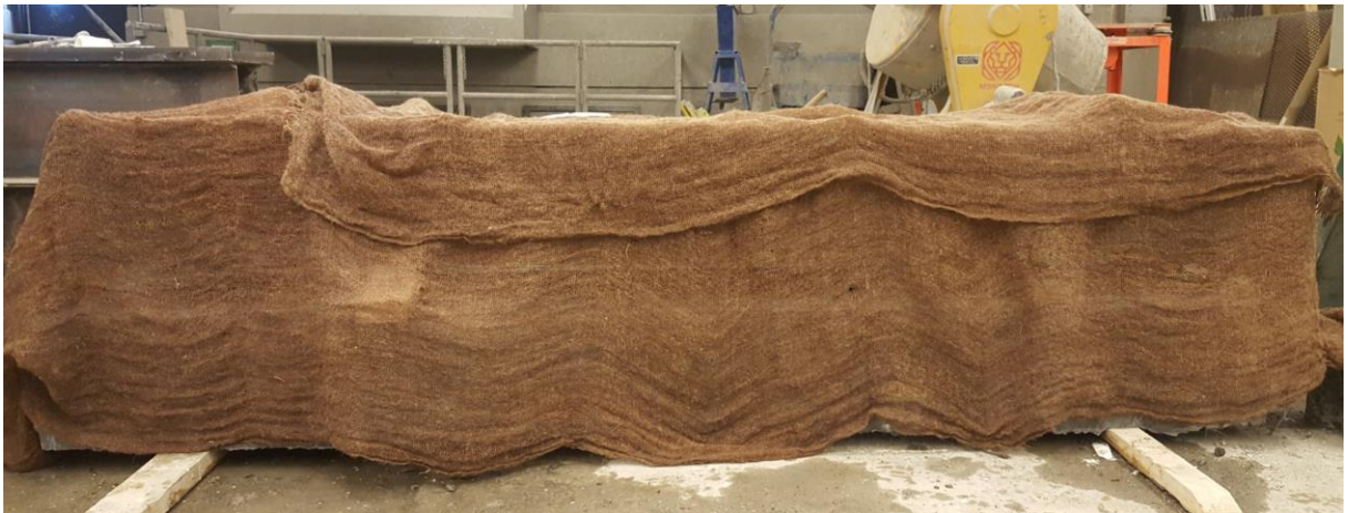
Figure 3-17 Curing of beams
