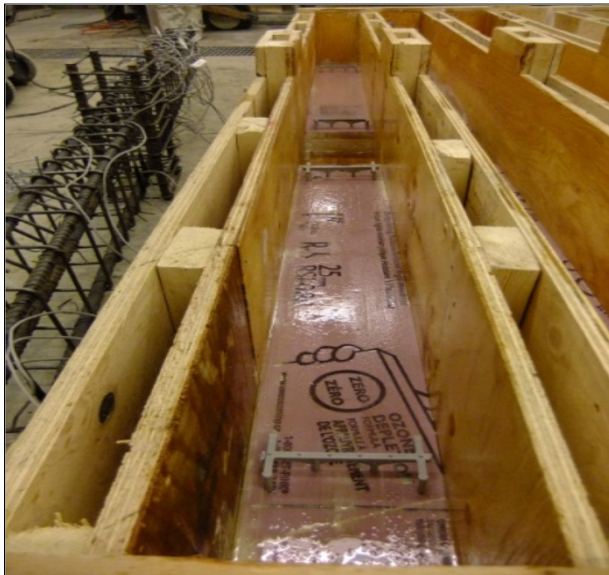
Figure 3.11 Reinforcement chairs and insulation foam used in formwork prior to casting
