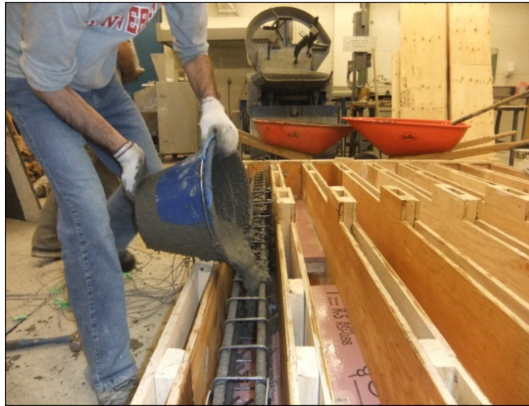
Figure 3.12 Casting beam D/2-0.0%
