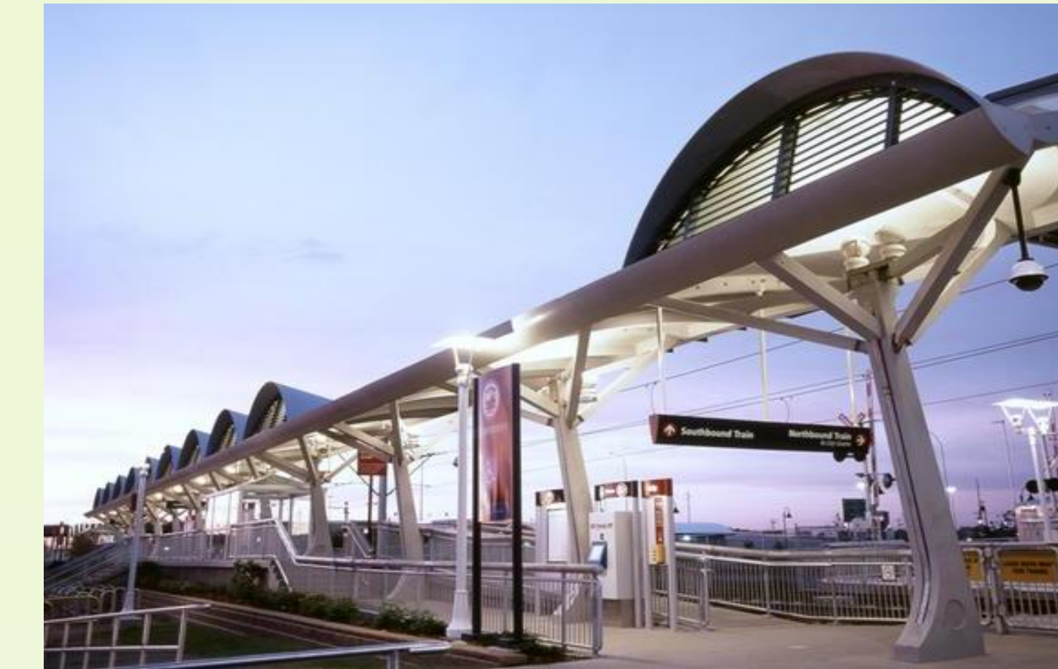
Figure 3: The Shawnessy Light Rail Transit (LRT) Station
