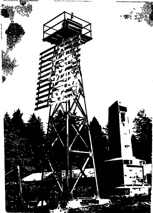
Fig. 24. On-shore range mark, ranging the first course of the International Boundary in the Gulf of Georgia. To the right is the monument marking the western terminus of the 49th parallel land boundary, erected in 1861 at a cost of nearly 1500.
