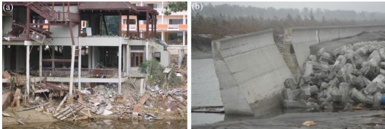
Figure 1.3: Tsunami damaged structures. (a) Building in Phuket Island, Thailand; (b) Breakwater in Natori, Japan (adapted from Esteban et al. (2015)).
