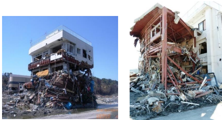
Figure 7.1: Debris impact on structures following the 2011 Tohoku Japan Tsunami (Nistor, 2011).
