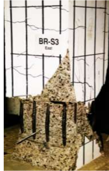
Column BR-S3 after test
