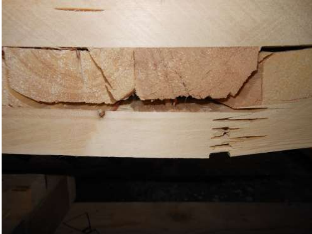
Figure 4.2: Finger Joint Separation in Tension Laminates
