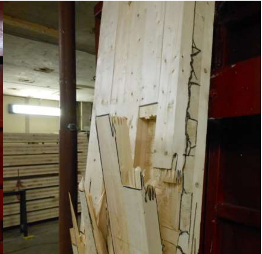
(b) Separation of Finger Joints - Right Side
