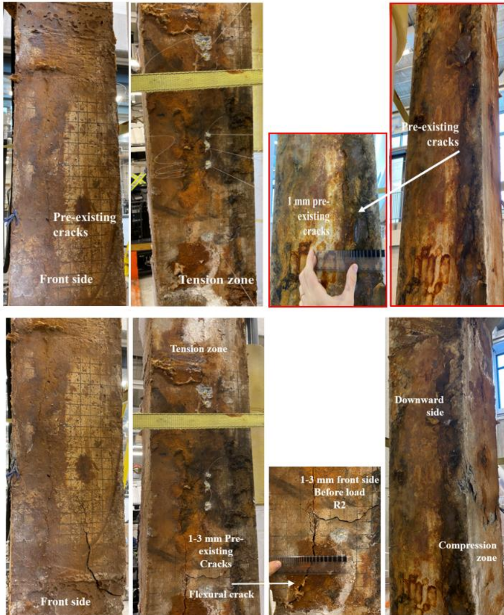
Fig. 5.6: Damage after loading for specimen C-E-R2
