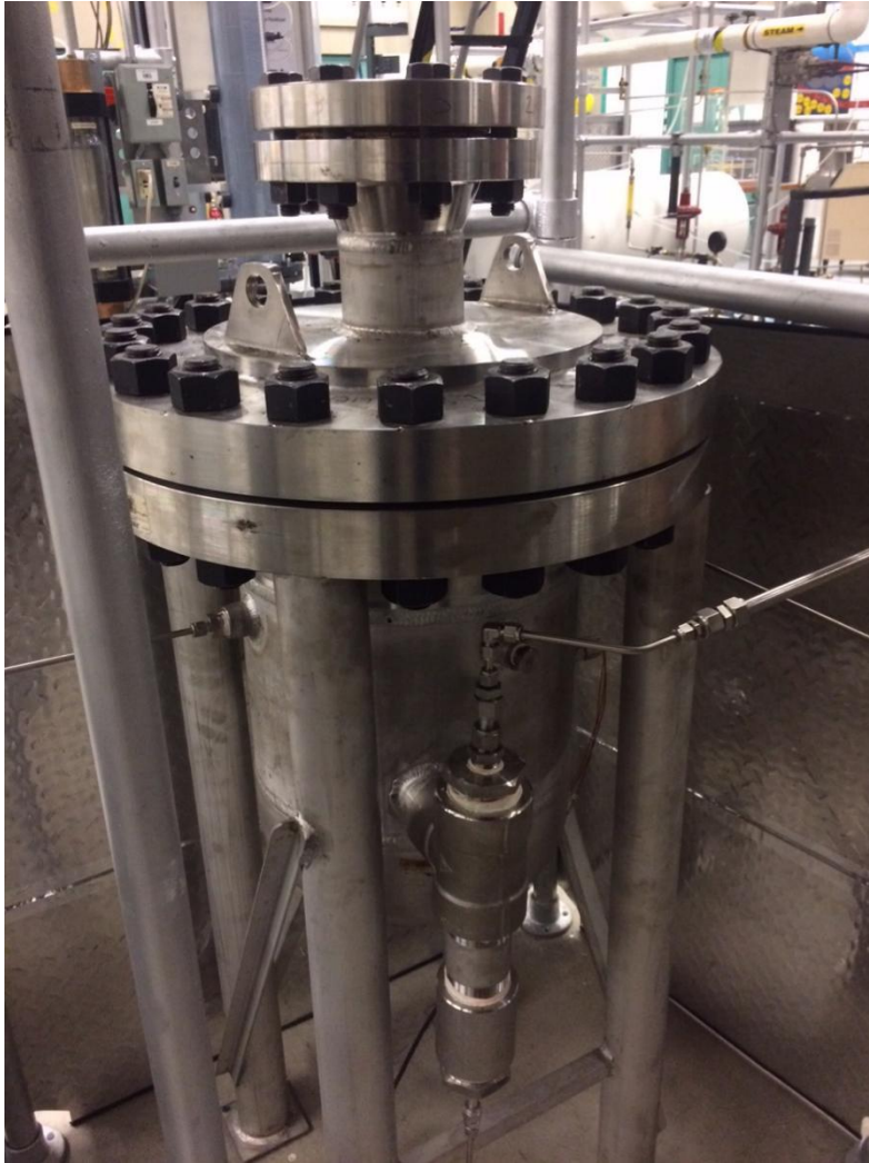
Figure A.2. View of the pressure vessel containing the feeder. The outlet tee has the auger pushing out the solids horizontally with the pneumatic convey gas coming from the top.
