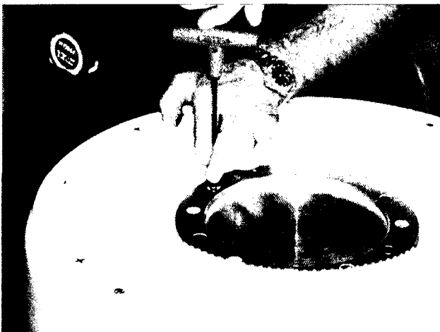
Figure 3.3 Steel base of the column open to cold room temperature
