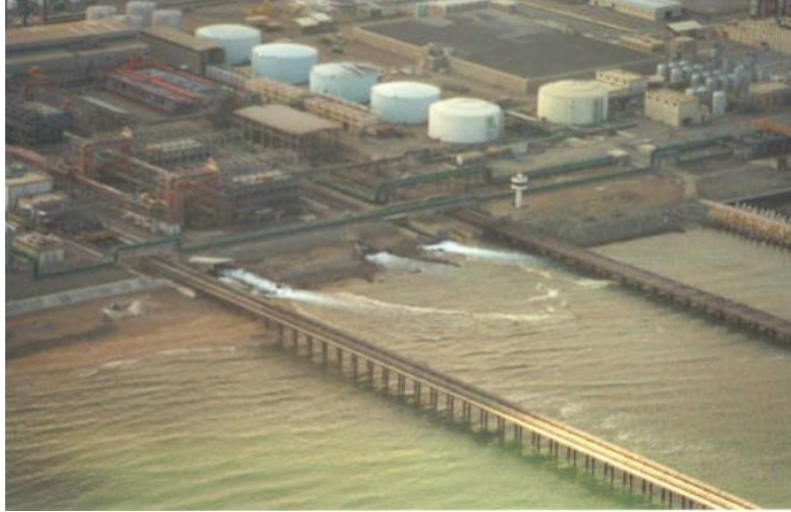
Figure 3.1: Al-Ghubrah desalination plant (largest in Oman) with a surface discharge (photo: H.H. Al-Barwani)
