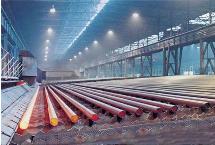
Fig. 1.7: A cooling bed for pipes (Photo from VMTubes 2009)
