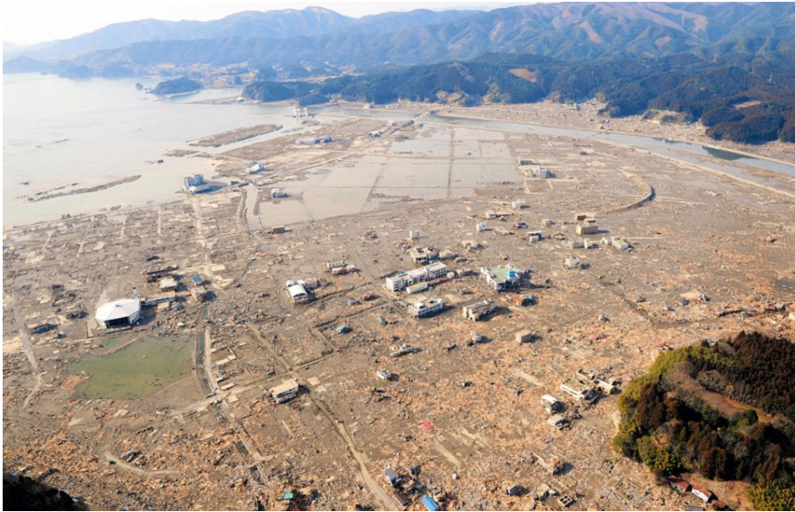
Figure 1.1 Photograph of the damaged endured in Rikuzentakata, Japan following the 2011 Tohoku earthquake and tsunami (Hagen 2014)
