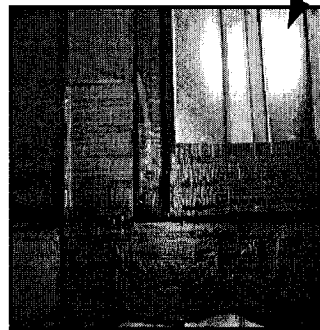
Edge treatment of the steel deck and L-channel
