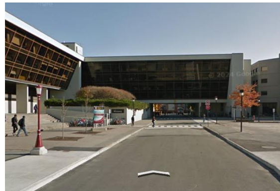
Figure 3.4 West Facing Wall
