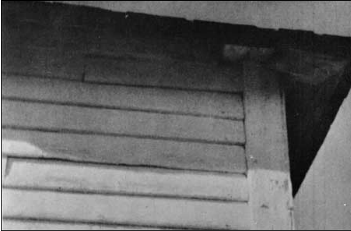
Figure 21. The technique of applying the weatherboarding and its attendant corner boards is well illustrated by a photograph of corner details on an 1830's building at Norway House. John A. Hussey. Fort Vancouver Historic Structures Report, Historical Data, Volume 1, June 1972. U.S. Department of the Interior.
