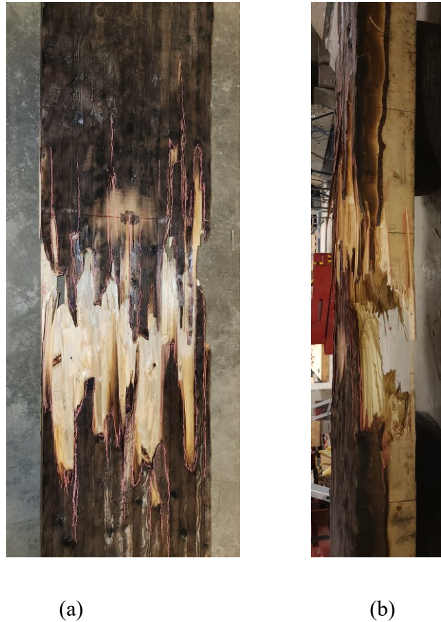
Figure 4-32 Dynamic Failure of CGLT7 [215] second shot: (a) After test - front view; (b) After test - side view
