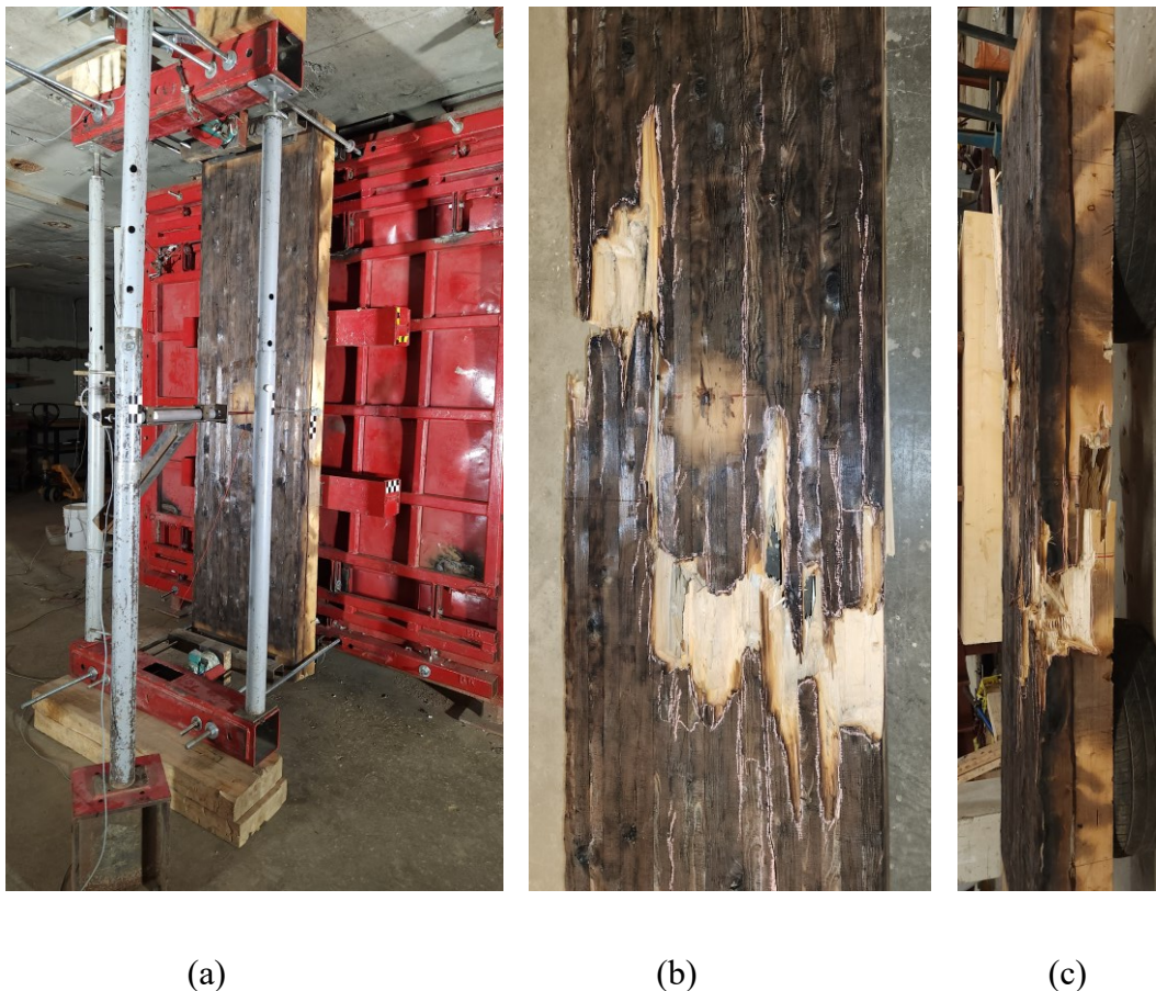
Figure 4-29 Dynamic Failure of CGLT5 [215]: (a) Before test; (b) After test - front view; (c) After test - side view
