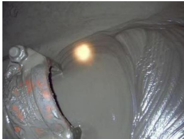
Figure 2.6 Sample of hydraulic backfill (Mohammad Pour, 2020).
