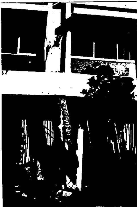
Figure 1.6: Ductile behaviour of a spiral column during the 1971 San Fernando Earthquake (Bertero 1985).
