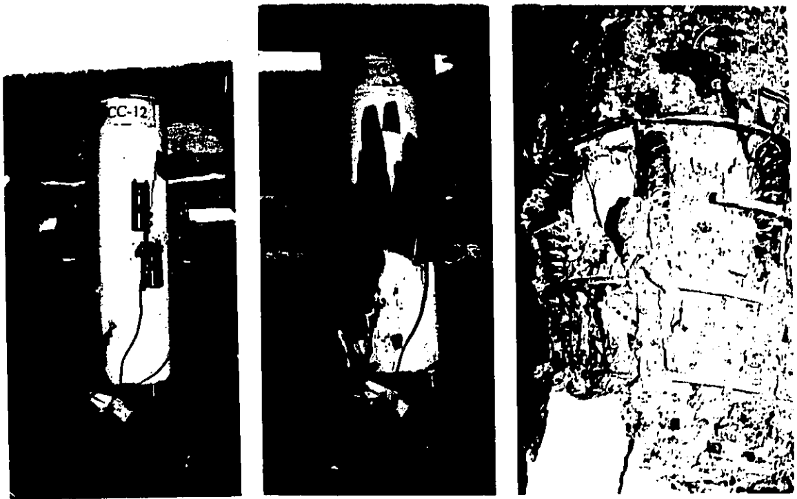
(b) Column behaviour during different stages of loading.
