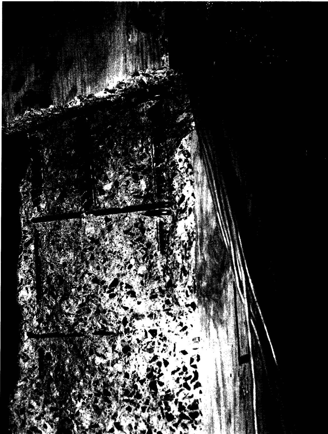
Figure 4.53: Significant concrete cover spalling in column at 1.75% lateral drift (BL-3)
