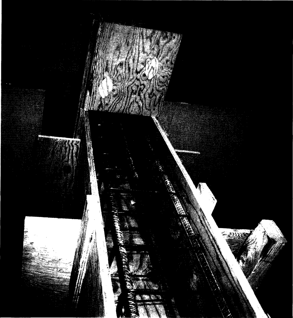
Figure 3.13: Reinforcement for top beam
