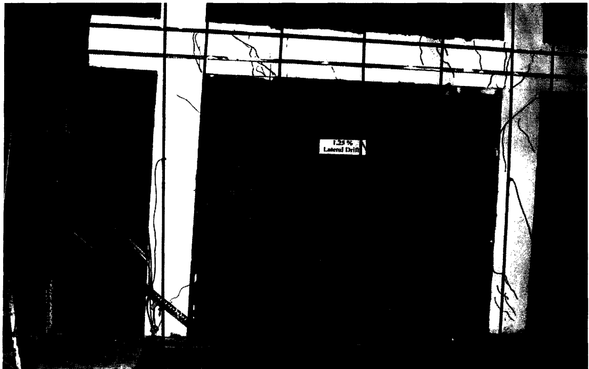
Figure 4.8: Crack pattern in specimen BR-1 at 1.25 % lateral drift
