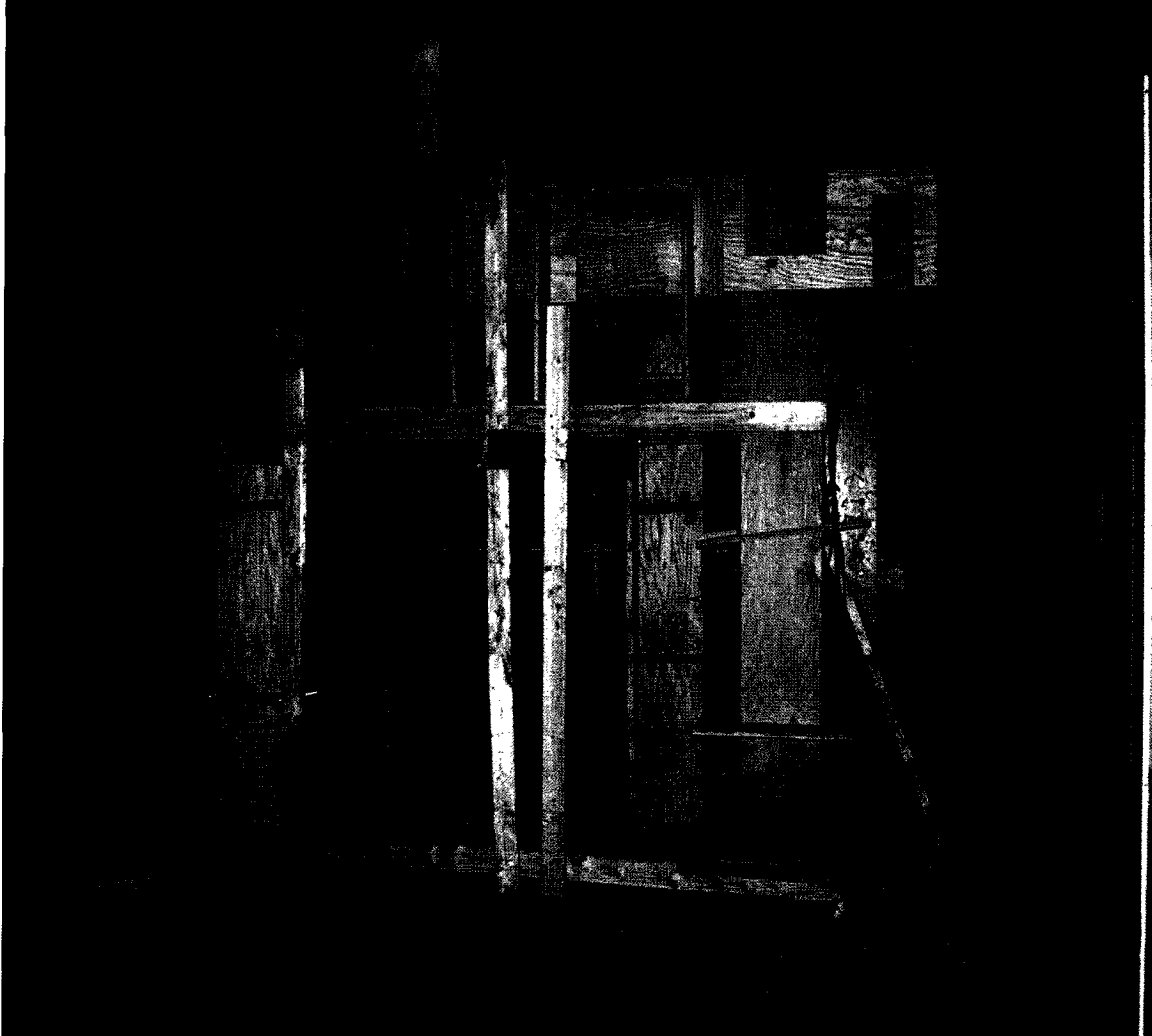
Figure 3.12: Complete frame formwork
