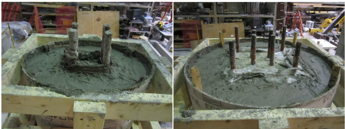
Figure 2-20 Third layer of concrete raiser units after concrete casting
