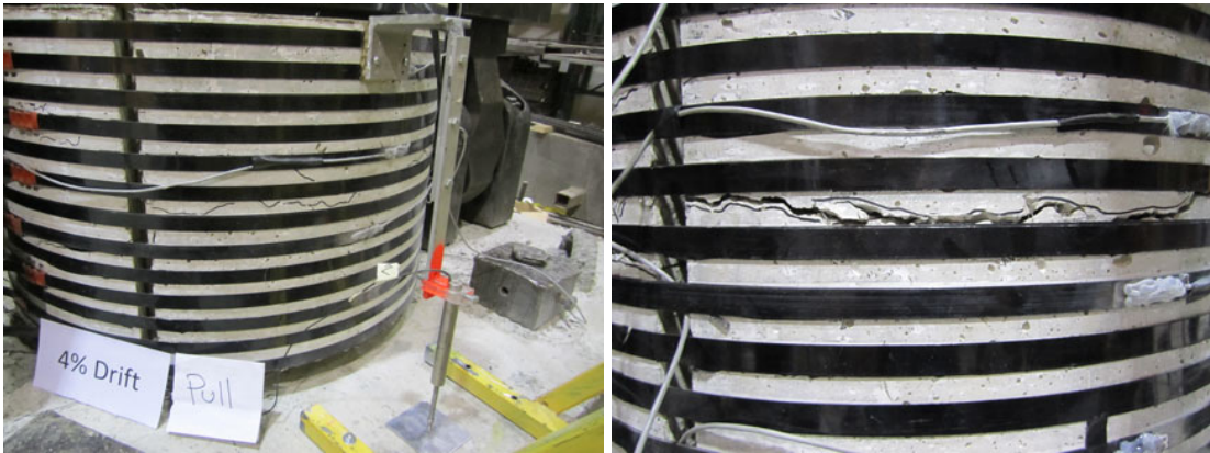
Cracks of the concrete raiser units after 4% drift
