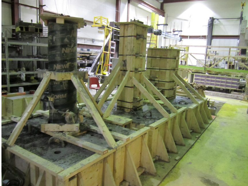
Figure 2-8 Column formwork after casting
