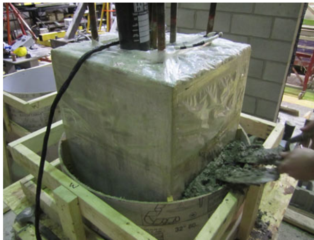
Figure 2-19 Placement of plywood on top of the first layer, and casting of the second layer
