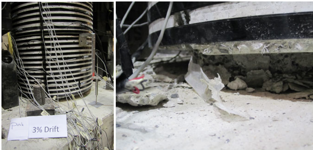
Delamination of main column at column-footing location after 3% drift
