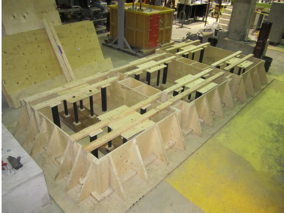
Figure 2-4 Footing formwork
