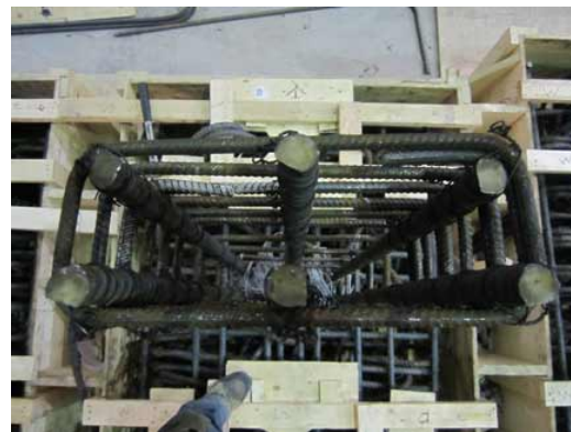
Figure 2-7 Column reinforcement cages
