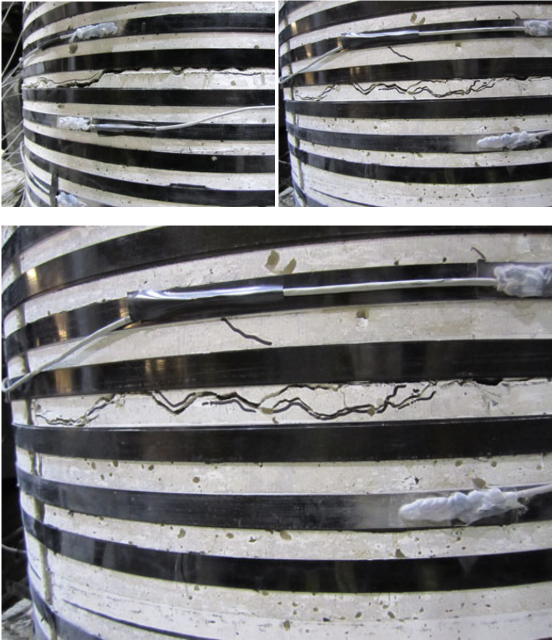
Figure 3-21 Rupture of 4 th strap and development of new cracks on the concrete raiser units after 6% drift
