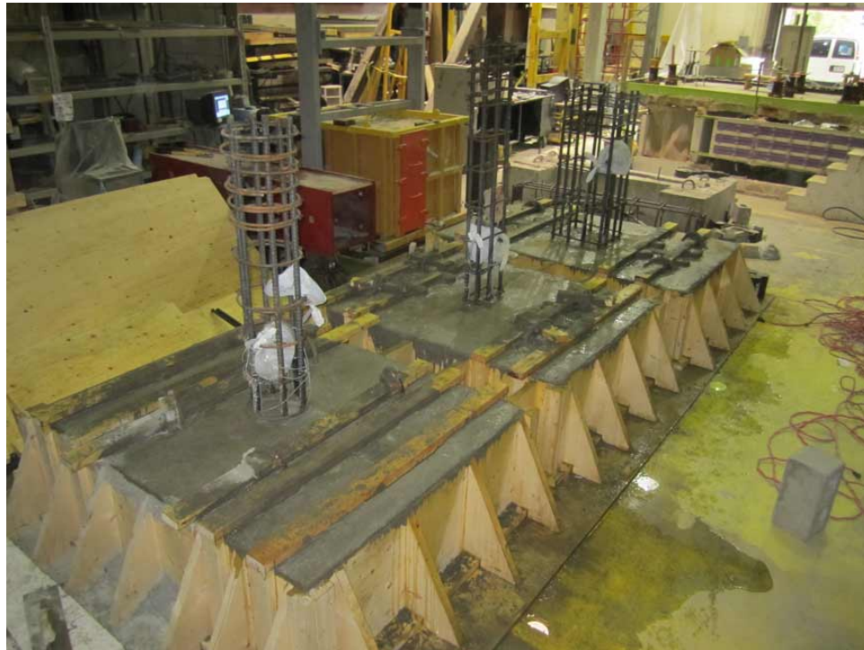
Figure 2-6 Footings after concrete casting
