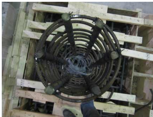
Figure 2-7 Column reinforcement cages
