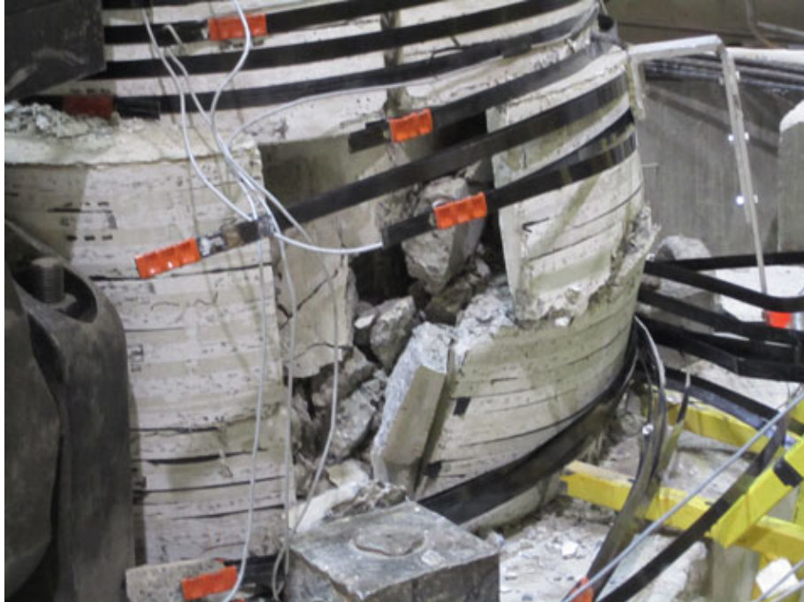
Failure of the column at second push at 7% drift
