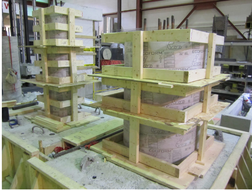
Figure 2-17 Concrete raiser unit formwork built around columns
