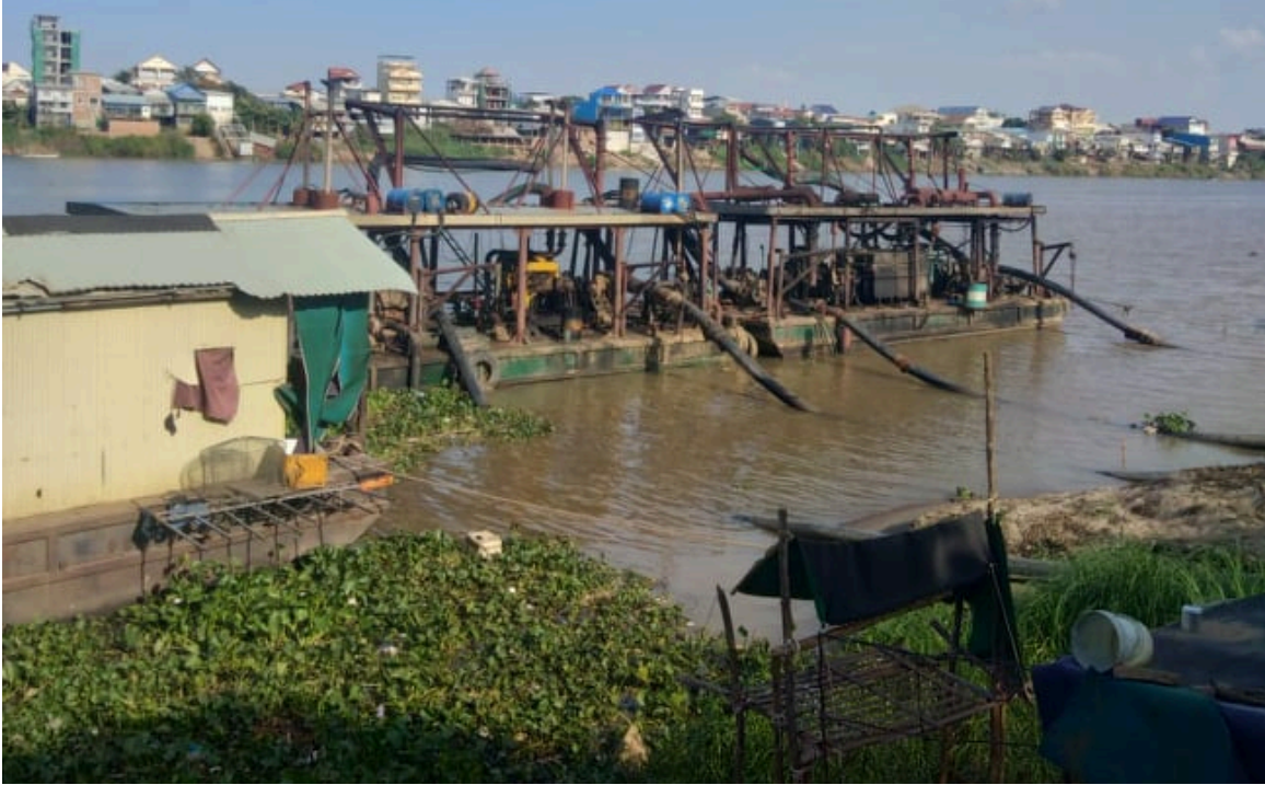
Figure 6.6 Sand pump station on the Mekong River, near Phnom Penh. The yellow raft left is the workers' living quarters.
