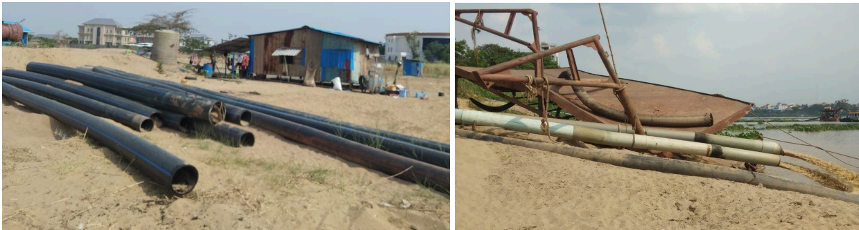
Figure 6.7 Unassembled sand pipes (left) and sand being pumped into wetlands for land reclamation purposes (right). See section 3.2.3.
