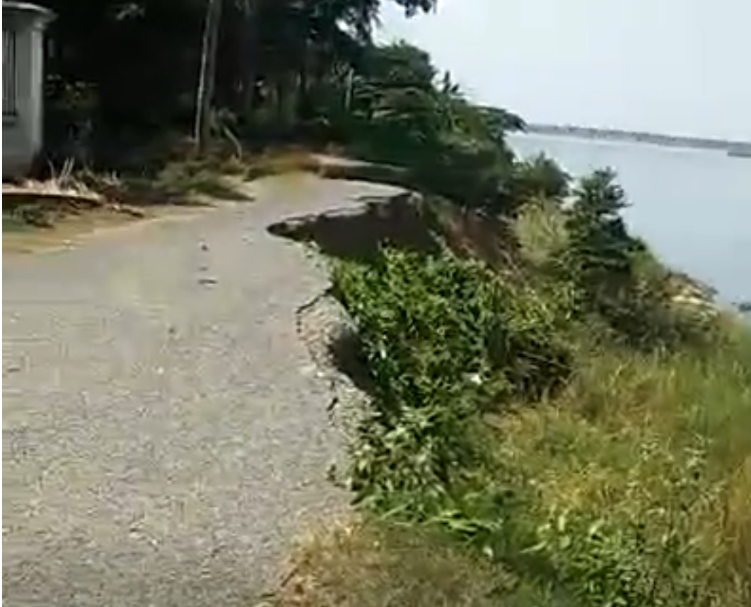
Figure 6.10 Snippet of a video taken by Munny showing an eroded road by the Mekong River.
