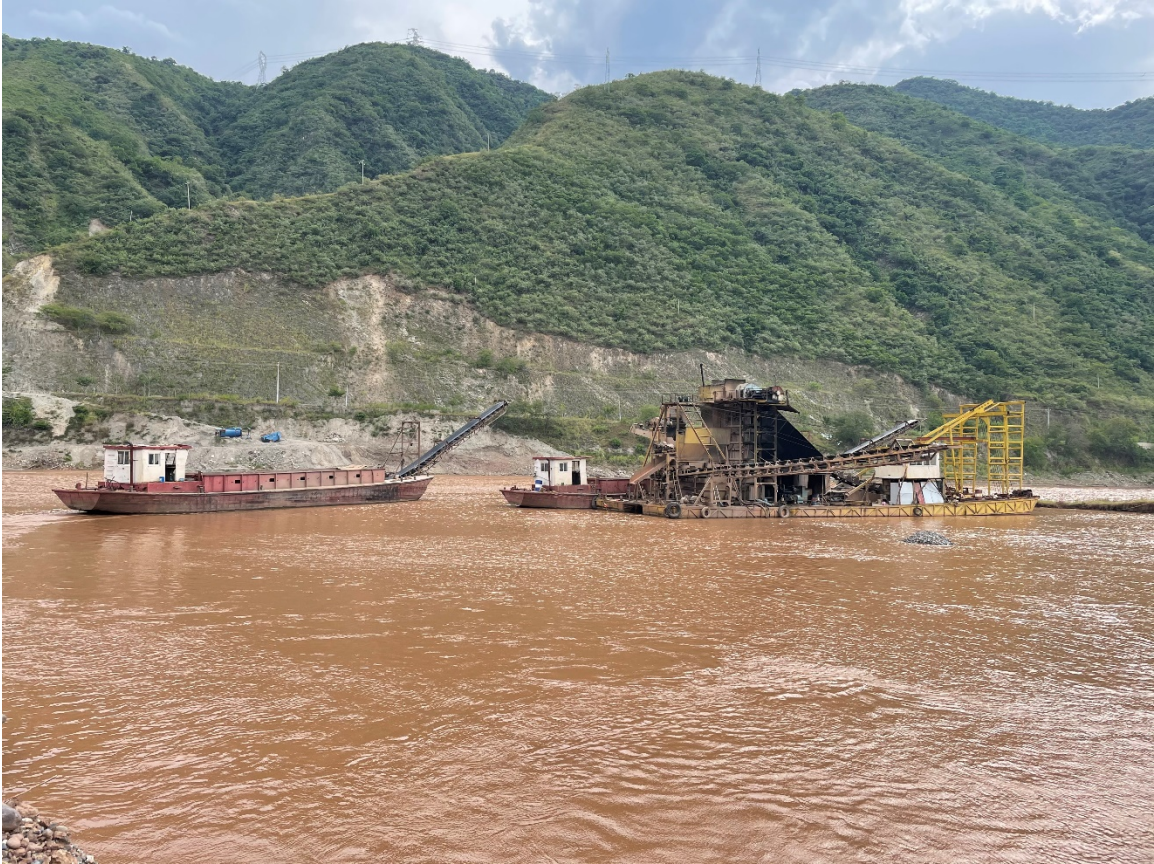
Figure 5.6 Two barges and a dredge on the Red River.
