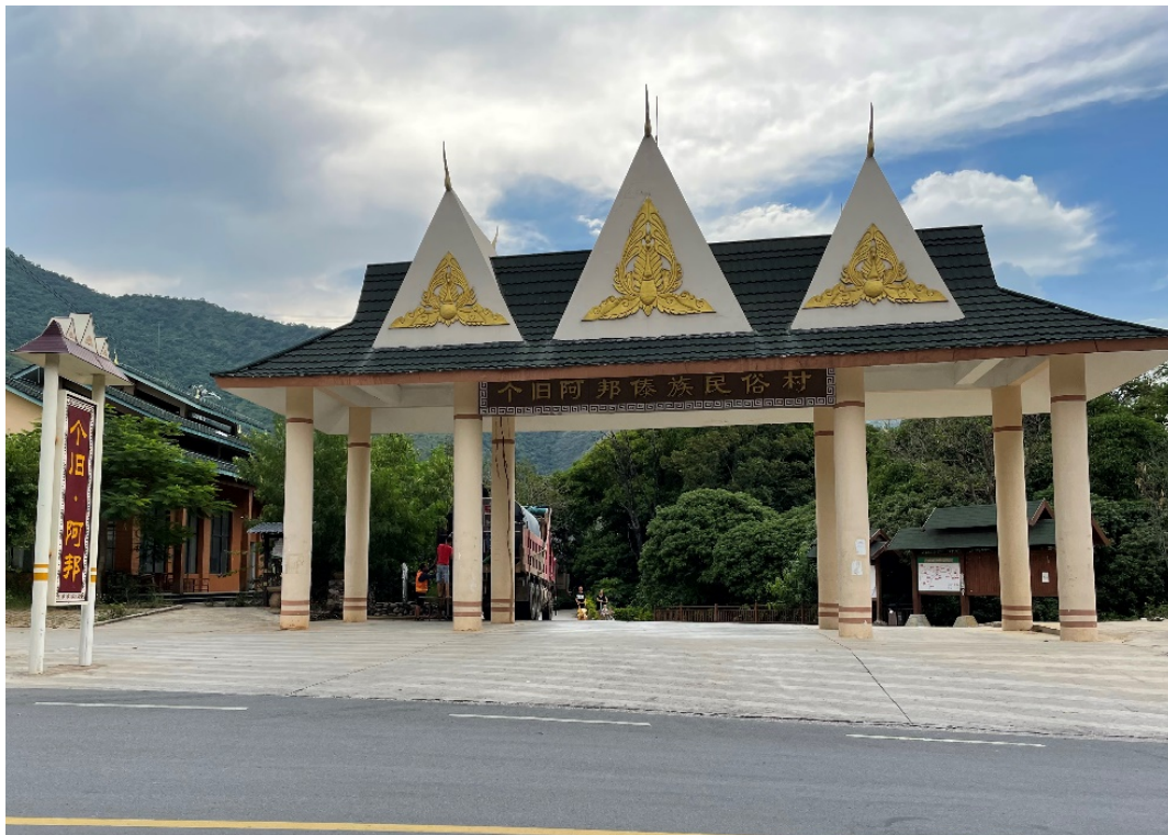
Figure 5.1 Gate built in village B by the government in the Folk destination remodeling.
