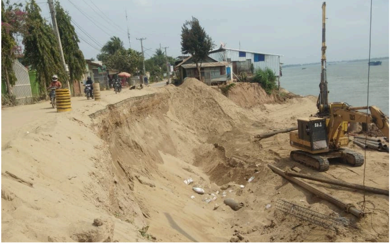
Figure 6.11 Eroded bank getting prepared for structural reinforcement.
