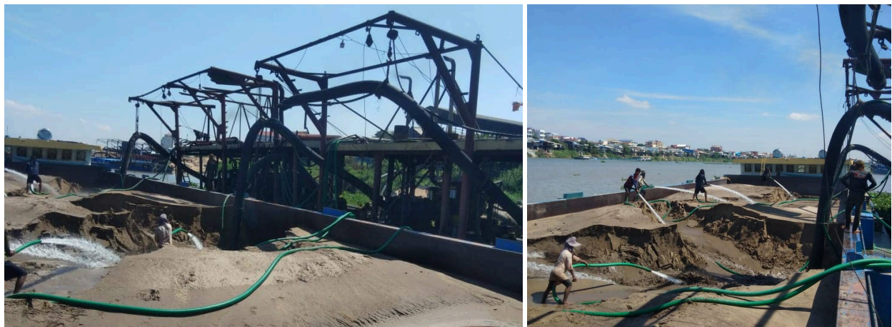
Figure 6.5 Sand labourers watering down sand in a barge to allow suction into the pipelines.
