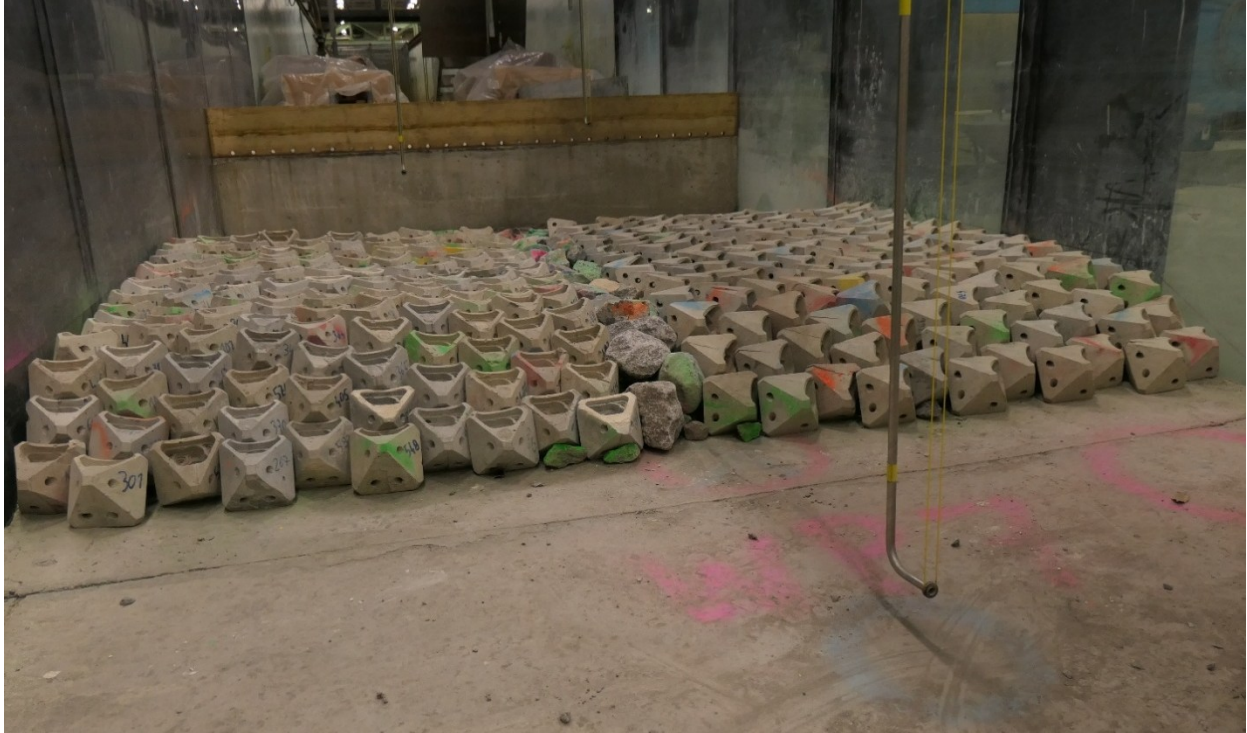
Fig. A3. Eco-friendly submerged breakwater case (TSCC) view no.2
