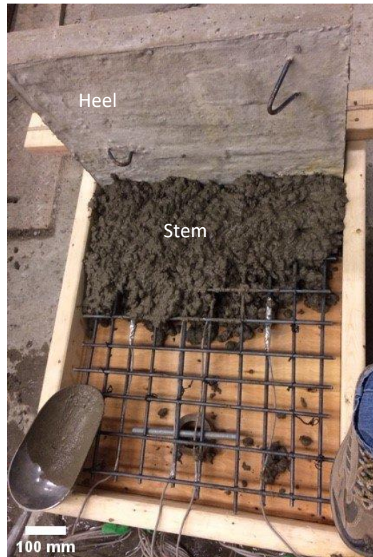
Figure 4.2: Reinforced concrete retaining wall Shown in the image is the process of casting for the stem. The heel of the retaining wall had already been cast.
