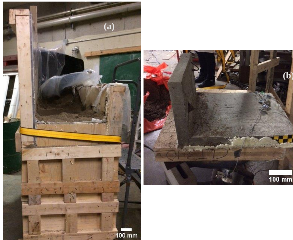
Figure 3.8: Wall removal and box disassembly after the test with loose backfill condition (a): front view of the test specimen after the removal of the RW and a portion of the box. (b): The RW was left aside until the box and the foundation layer were fixed
