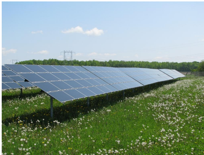
Figure 1.1: Arnprior solar plant, made out of 319 000 CdTe panels. Photo courtesy of Mark Yandt.
