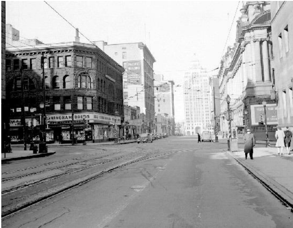
Fig. 9. Hastings Street, Vancouver. Intersection of Granville Street in foreground. (Image from Vancouver of the Mind .)
