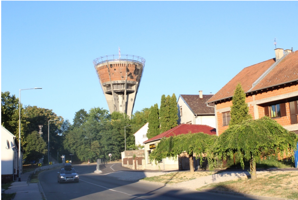
Figure 25: The water tower of Vukovar is a symbol of the town and its endurance during the siege. It was renovated so as to retain the evidence of the JNA shelling.
