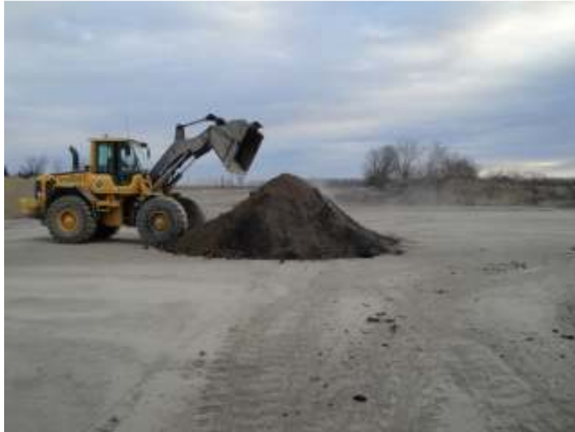
Photo B.1 Mixing Contaminated Soil with Compost Amendment
