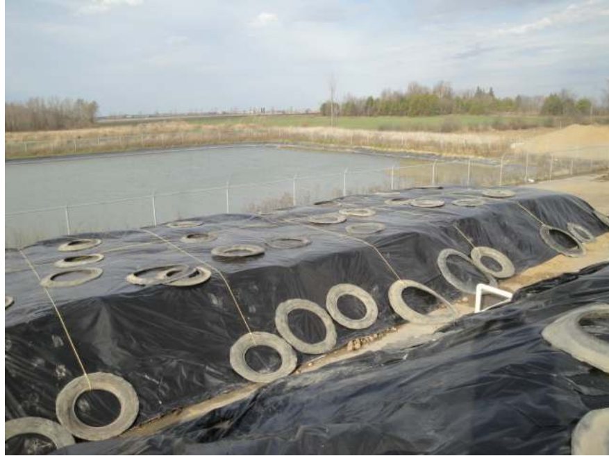
Photo B.5 Finished biopiles with black plastic cover
