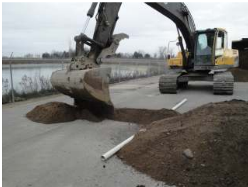
Photo B.2 Biopiles construction
