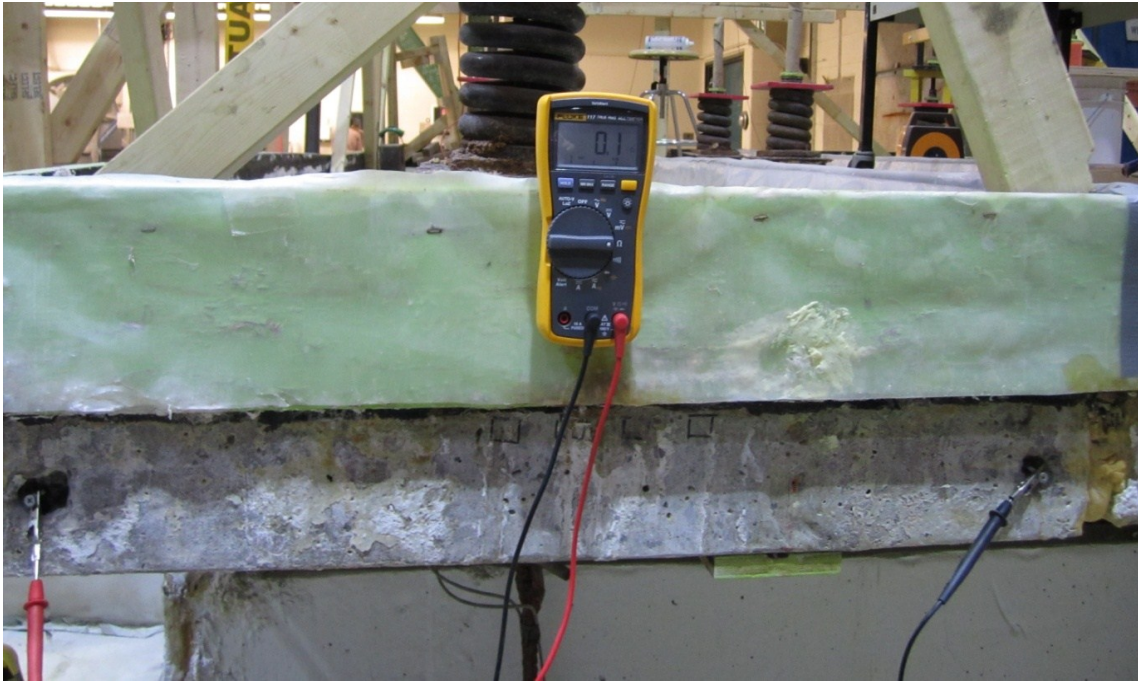
Figure 3-12: The electrical connection of the reinforcement was checked using the multimeter. The electrical resistance between the first and the last rebars was 0.1 Ohm.
