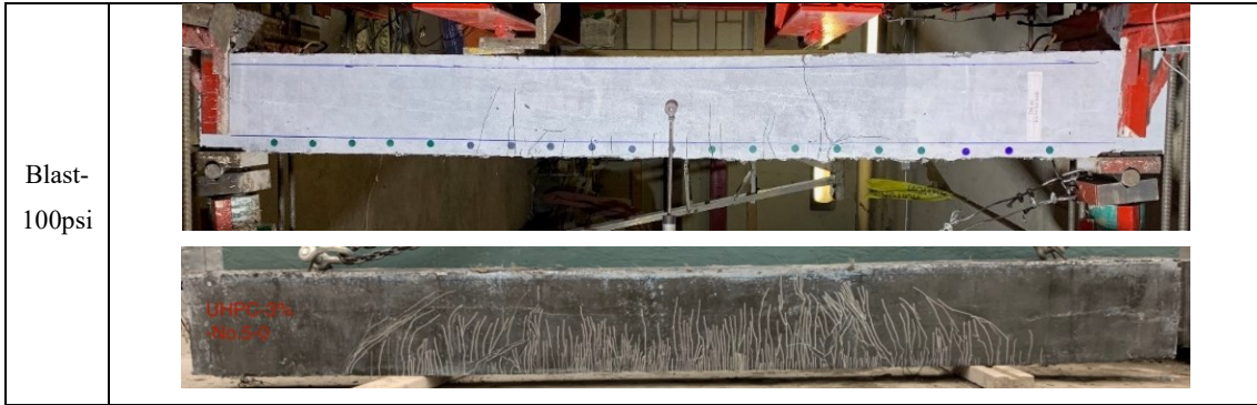
Figure A.125 Blast damage for beam U2-20M-DR-d/2
