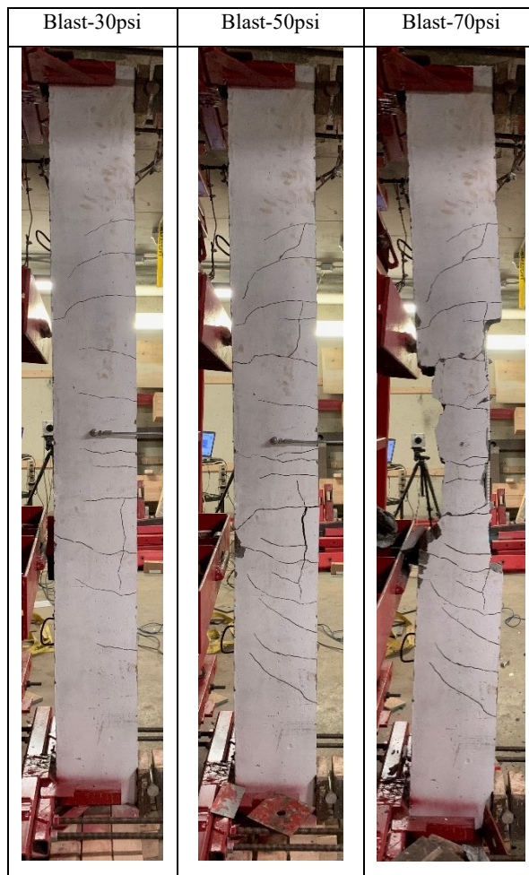
Figure A.72 Blast damage for beam C100-No.5S1-S
