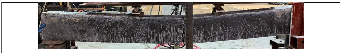
Figure A.111 Failure mode after the post-blast residual static test
