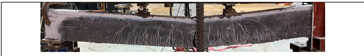
Figure A.123 Failure mode after the post-blast residual static test
