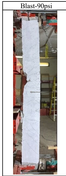
Figure A.65 Blast damage for beam C100-No.5HS-DR-d/4 (x1)
