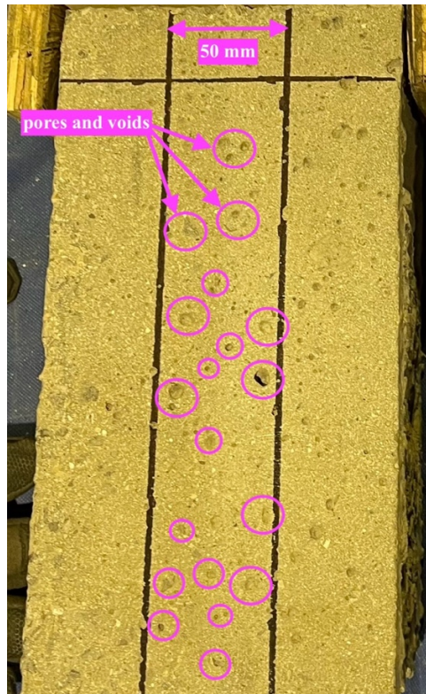
Fig. 5-42. Surface imperfections in the bond area of specimen HM-2 showing voids and cavities on the concrete substrate.
