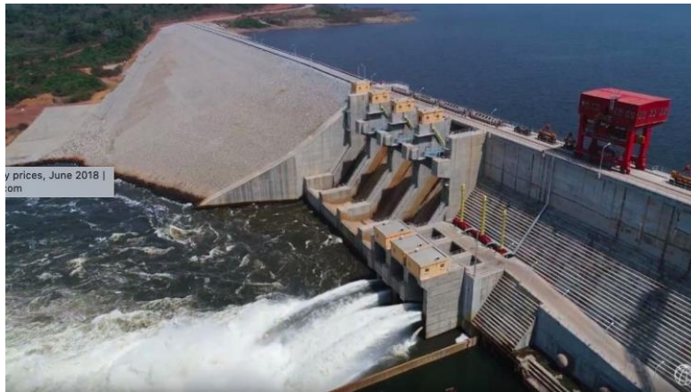
Figure 3.2: Lom Pangar Dam
