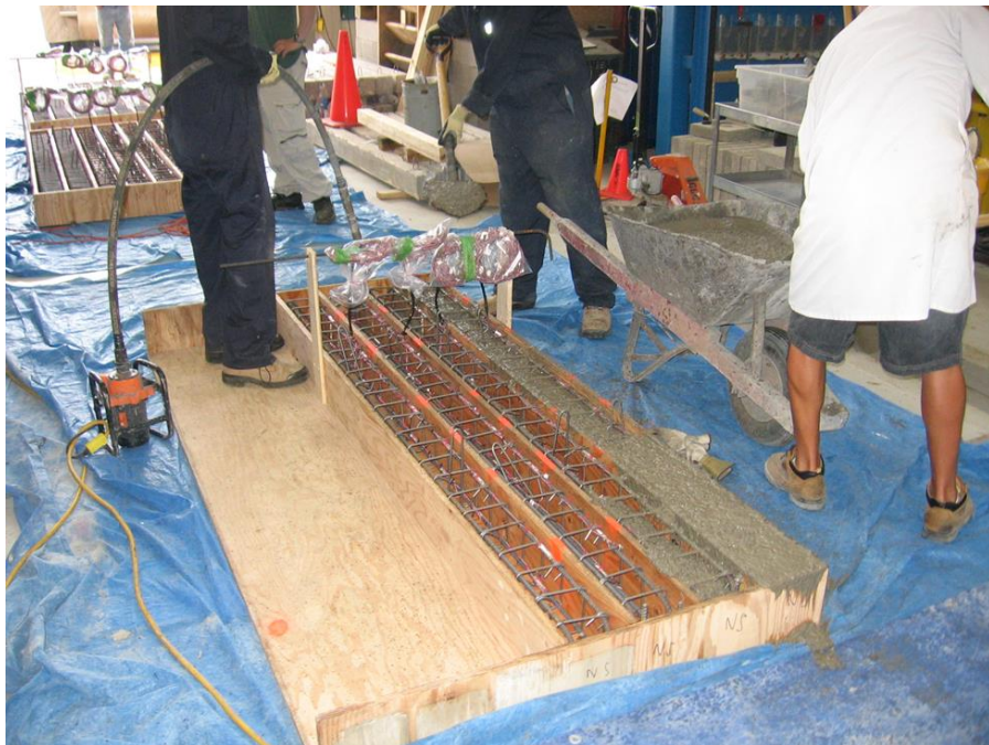
Fig. 3.6 Concrete vibration
