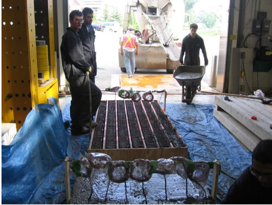
Fig. 3.5 Concrete supply and placement
