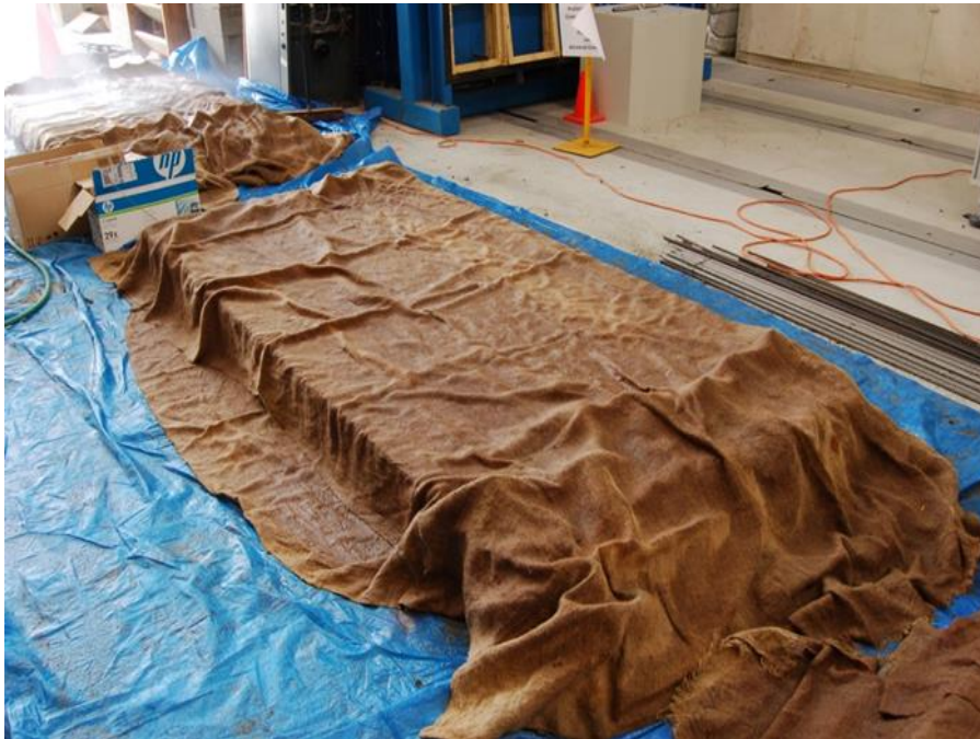
Fig. 3.8 Concrete curing by wet burlap
