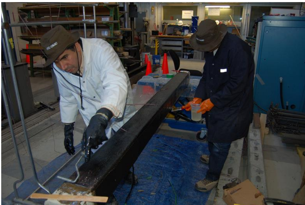
Fig. 3.14 Application of CFRP by wet-layup method
