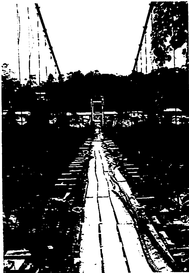
Photo 10: The suspended bridge over the Misahualli River at Pujillo
