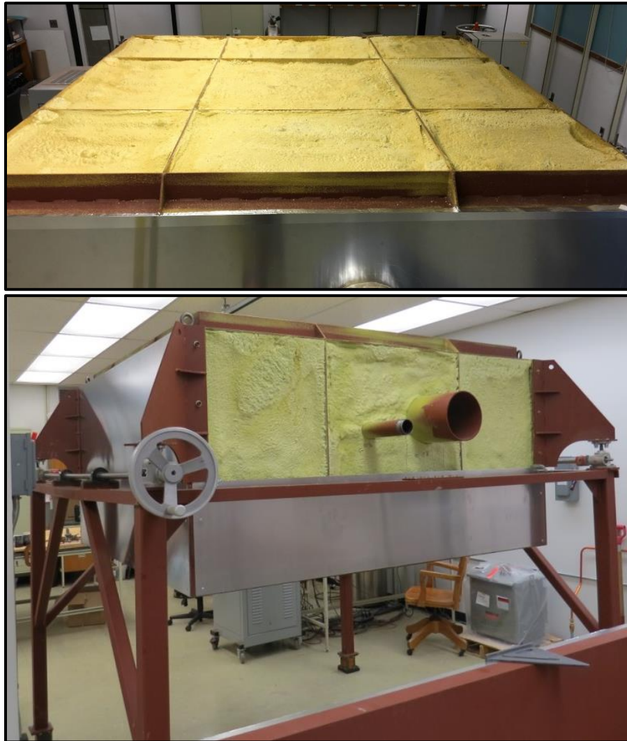
Figure 4-15: Insulating the Exterior Walls of the GHB
