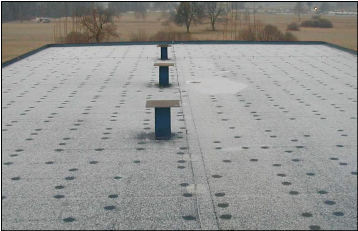
Figure 2-27: In-situ Fastener Thermal Impact (retrieved from Wieland, 2006)
