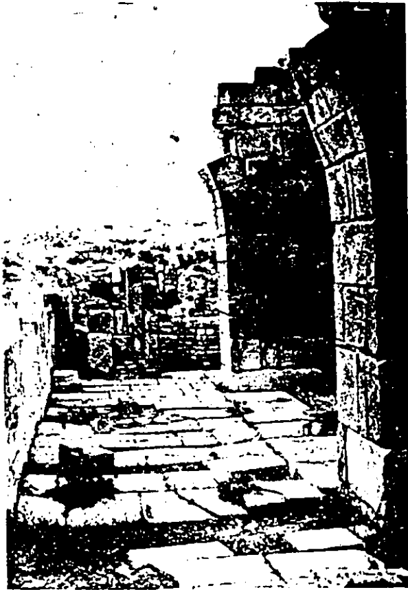
Fig. 3 Eastern face of supporting piers.
