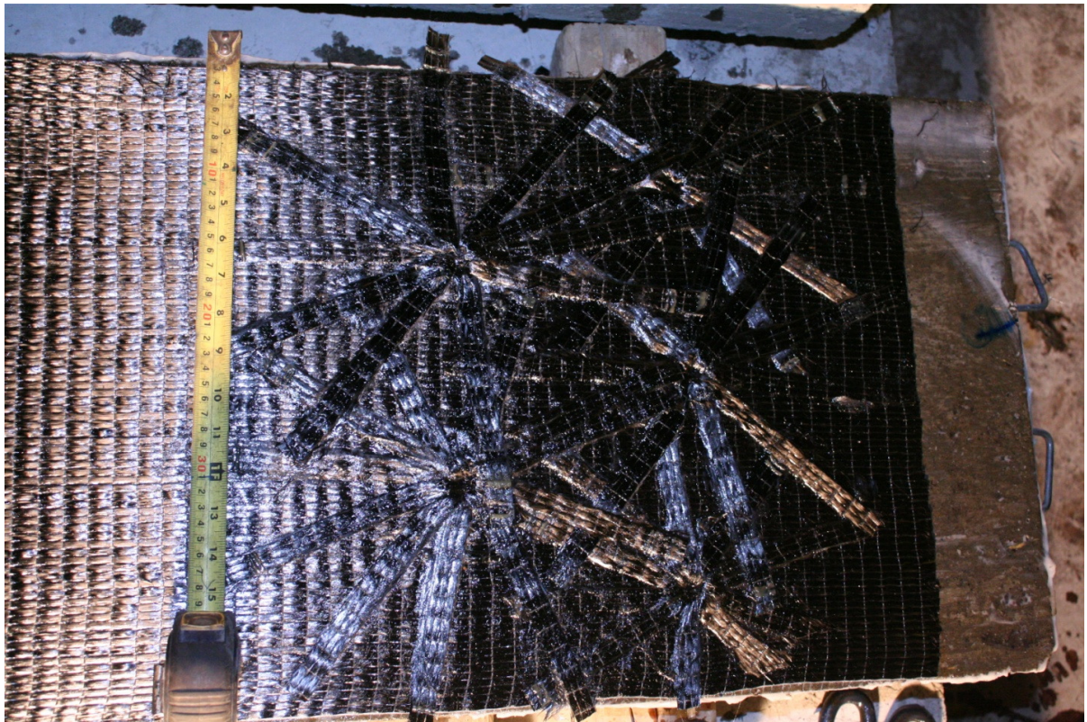
Figure 3.24: Typical FRP Anchor Placement.
