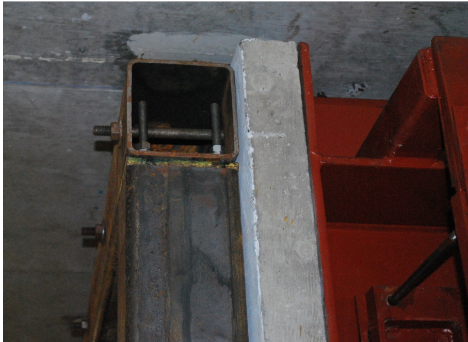
Figure 3.15: Close-up of Support Conditions for Companion Set 5.
