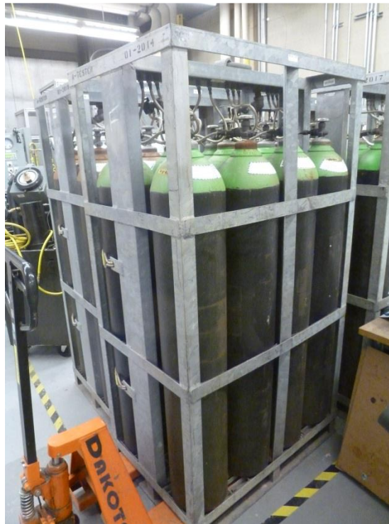
Figure 4.13: Nitrogen bottle reservoir (bottle pack).
