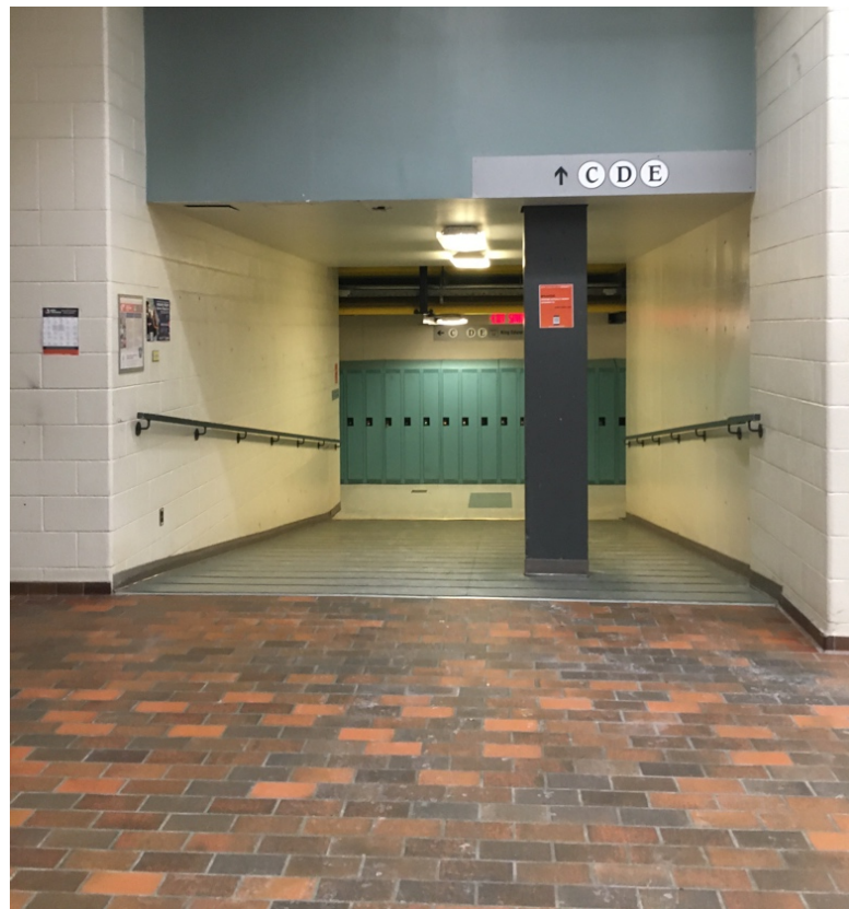
Figure 5-7 - CBY floor 0 ramp leading to block C, slope of 1:7.5
