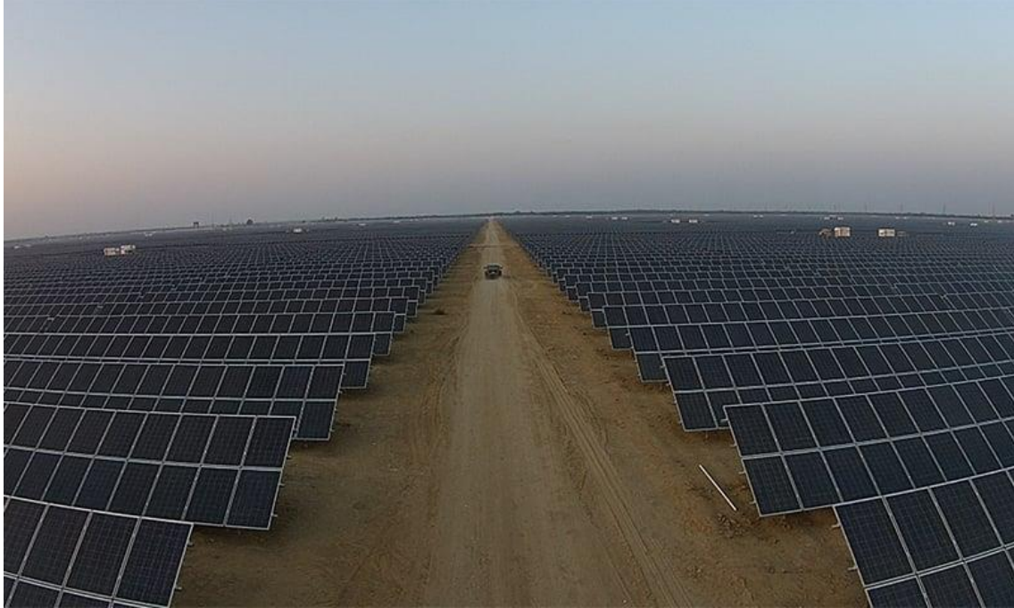
Figure 1.2 QASP solar system. Photo credit Quaid-e-Azam Solar Power (Pvt) Ltd. Retrieved from: https://www.dawn.com/news/1209933
