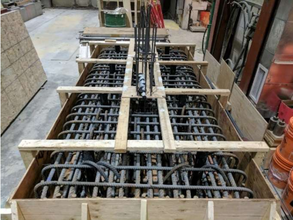
a) Wall W1HS foundation before casting
