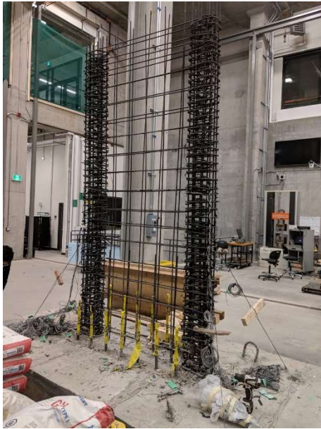
c) Wall W2HS prior to casting
