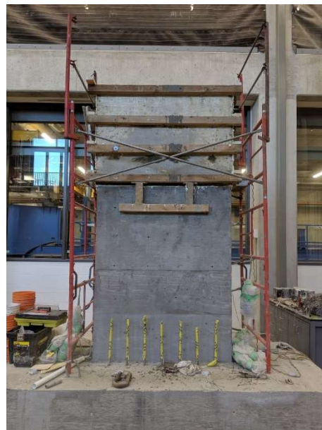
d) Wall W2HS – during casting
