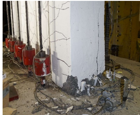
d) East side boundary element at test end
