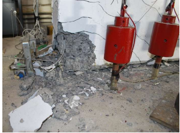
b) Crack at wall base at the end of testing
