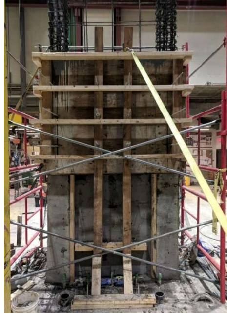
b) Wall W1HS – during casting
