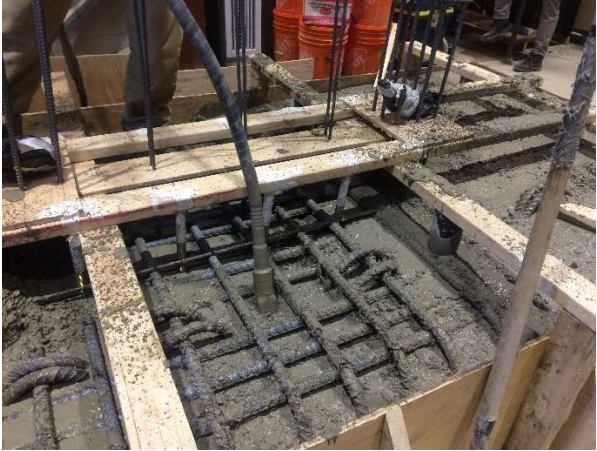
d) Wall W1HS foundation during casting
