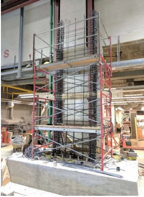
a) Wall W1HS prior to casting
