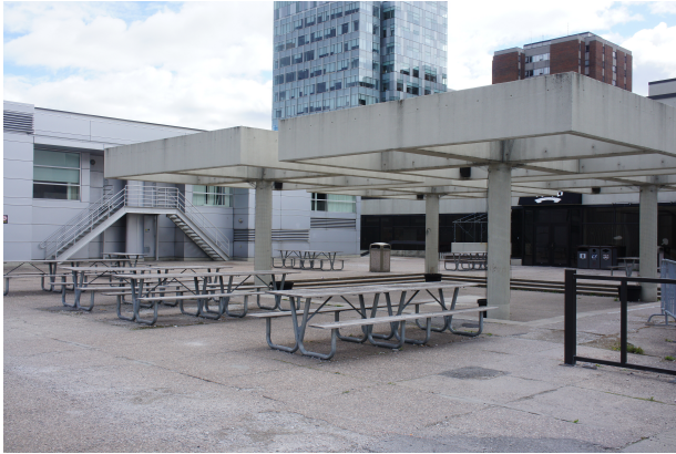
Figure 5: Courtyard at the University Centre
