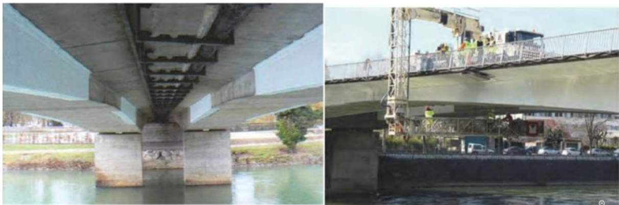
Figure 2.10 - In-situ Infrared bridge inspection a)View of strengthened regions (left), b) mounted lift-platform (right) (Taillade et al., 2012)
