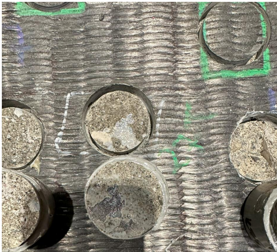
F.0.9 -Bond separation between layers in defective pull-off specimens
