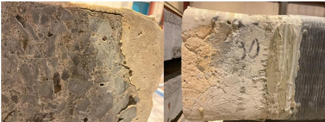
Figure 3.1-Cracks in patch materials
