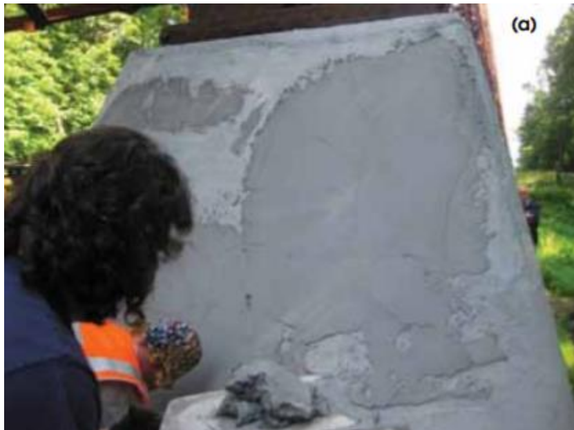
Figure 2-18: Preparing the substrate of pedestal ACI 549.4R-20).
