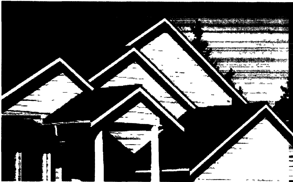
(a) Steep slope roof for residential house
