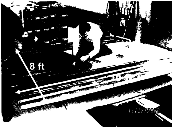
(a) Construction of a mock-up and curing with a specific time period
