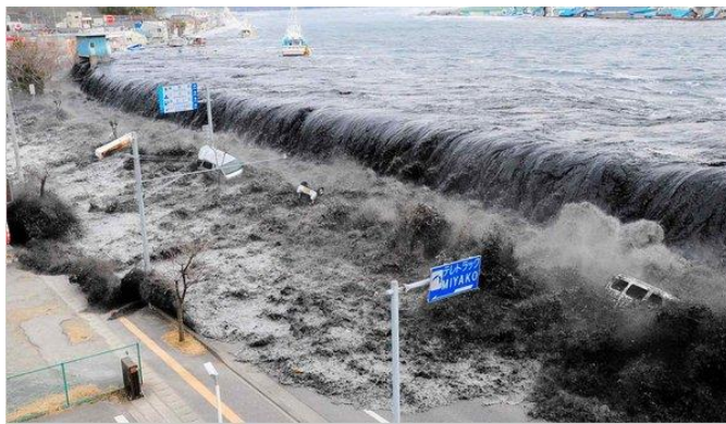
Figure 1.3 - Seawall overtopping in Miyako, Japan [Asahi Shimbun, 2010]
